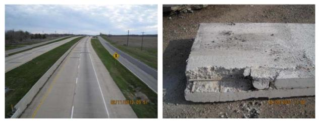
(a) Pavement Condition (b) Transverse Steel above Longitudinal Steel
