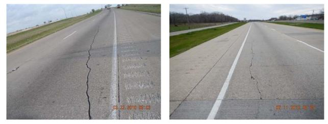
Figure 5.3 Longitudinal Cracking in CPCD Figure 5.4 Longitudinal Cracking in CRCP
