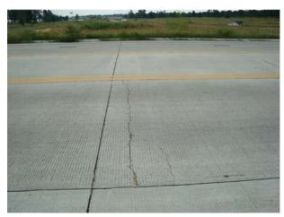
**Figure 5.1 Faulting in Transverse Joint**
