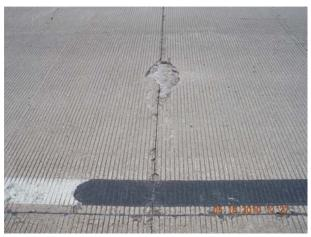
Figure 5.8 Spalling at Saw Cut Joint Due to Micro-Damage in Concrete
