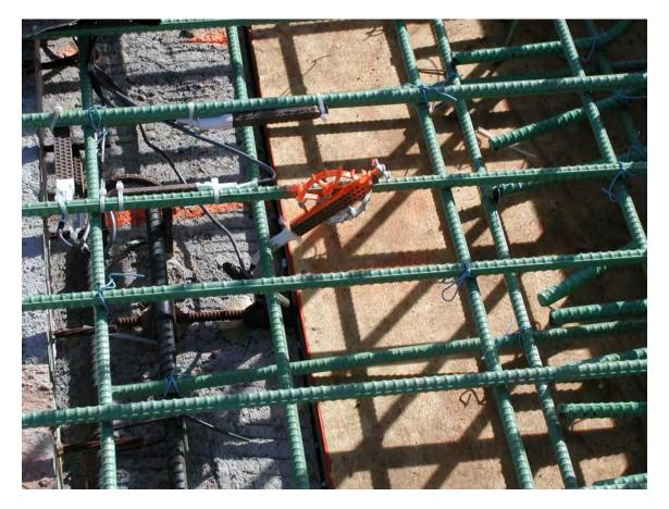
Figure 3.9 Embedded Strain Gauges at the Overhang of the Bridge Deck
