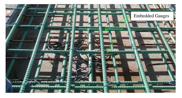
Figure 3.10 Embedded Gauges in the Controlled Joint Between Spans 1 and 2
