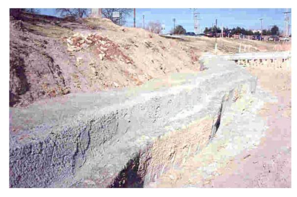
Figure 5.10 Partially Completed Retaining Wall Containing Tire Bales (NMED 1999)
