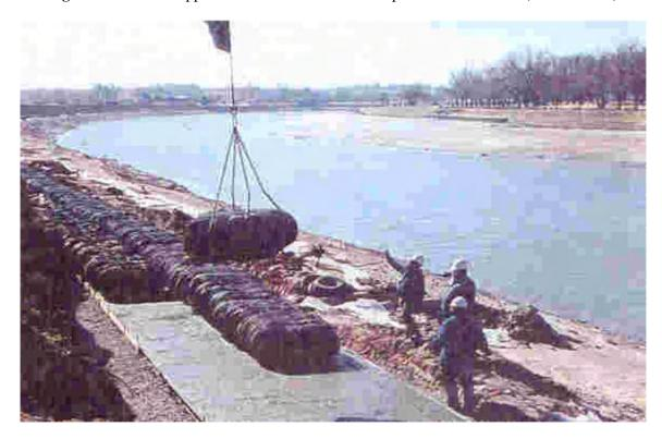
**Figure 5.8** Placement of One-Ton Tire Bales onto Concrete Base (NMED 1999)
