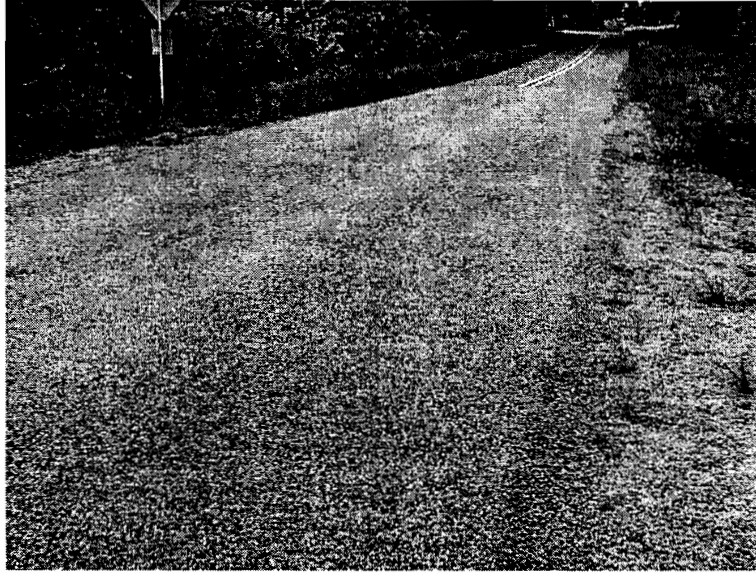
Figure 5.34 Pavement Section over Installation A1 in Atlanta District.
