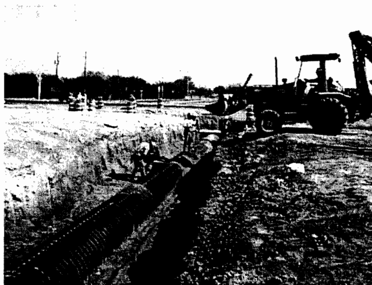
Figure 5.17 Backfill Placement and Compaction.
