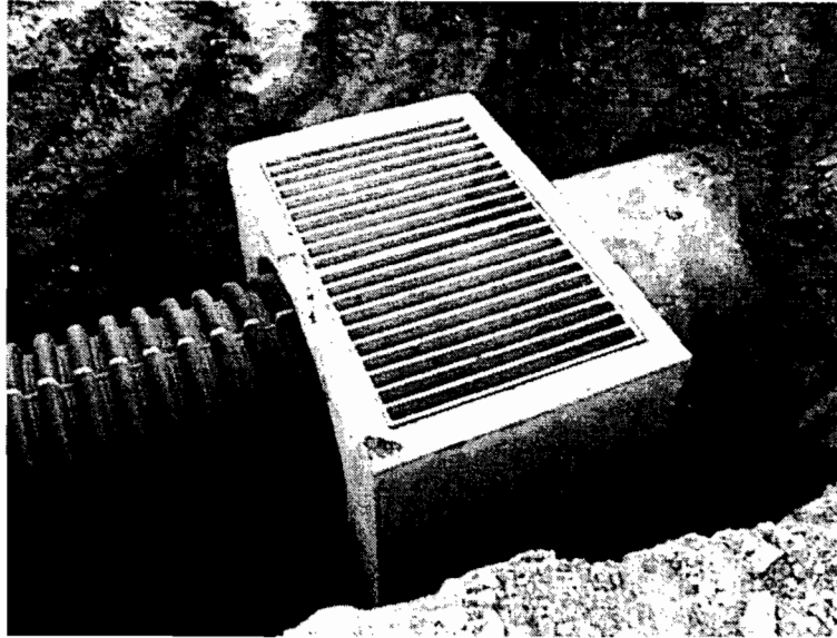
Figure 5.16 Existing Concrete Catch Basin and HDPE Pipe.
