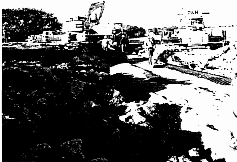
Figure 5.6 Pipe with Backfill up to the Crown.
