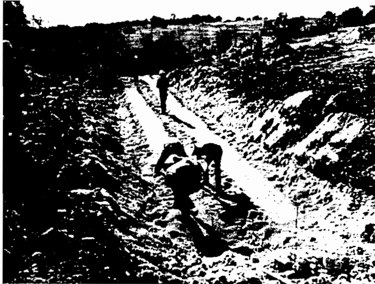
Figure 5.4. Shaping of the Bedding.
