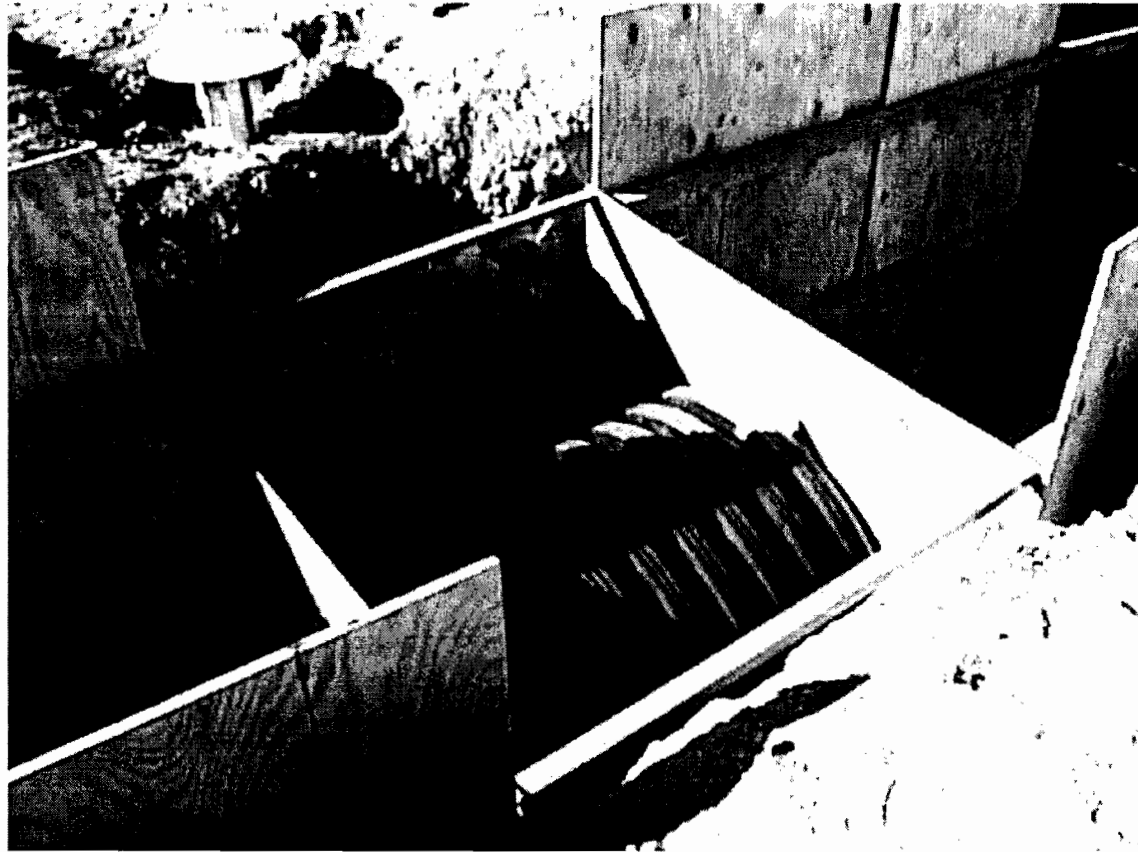
Figure 4.12. A Pipe Section Ready for the Placement of Backfill.
