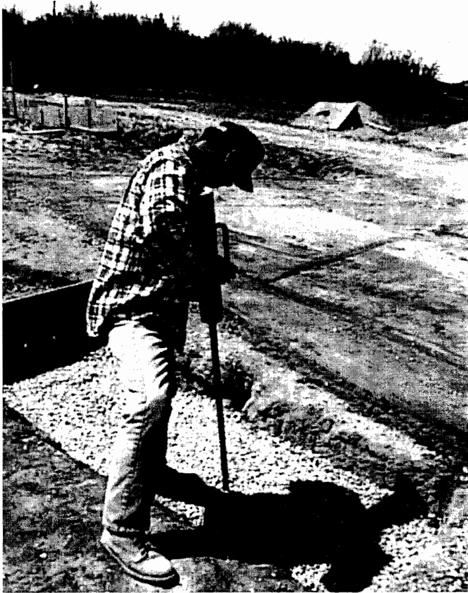
Figure 4.4. The Dynamic Cone Penetrometer Being Operated.
