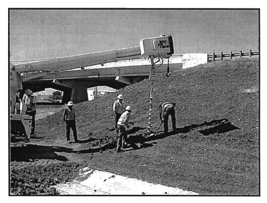
Figure 11. Drilling Boreholes at Motley Drive Site
