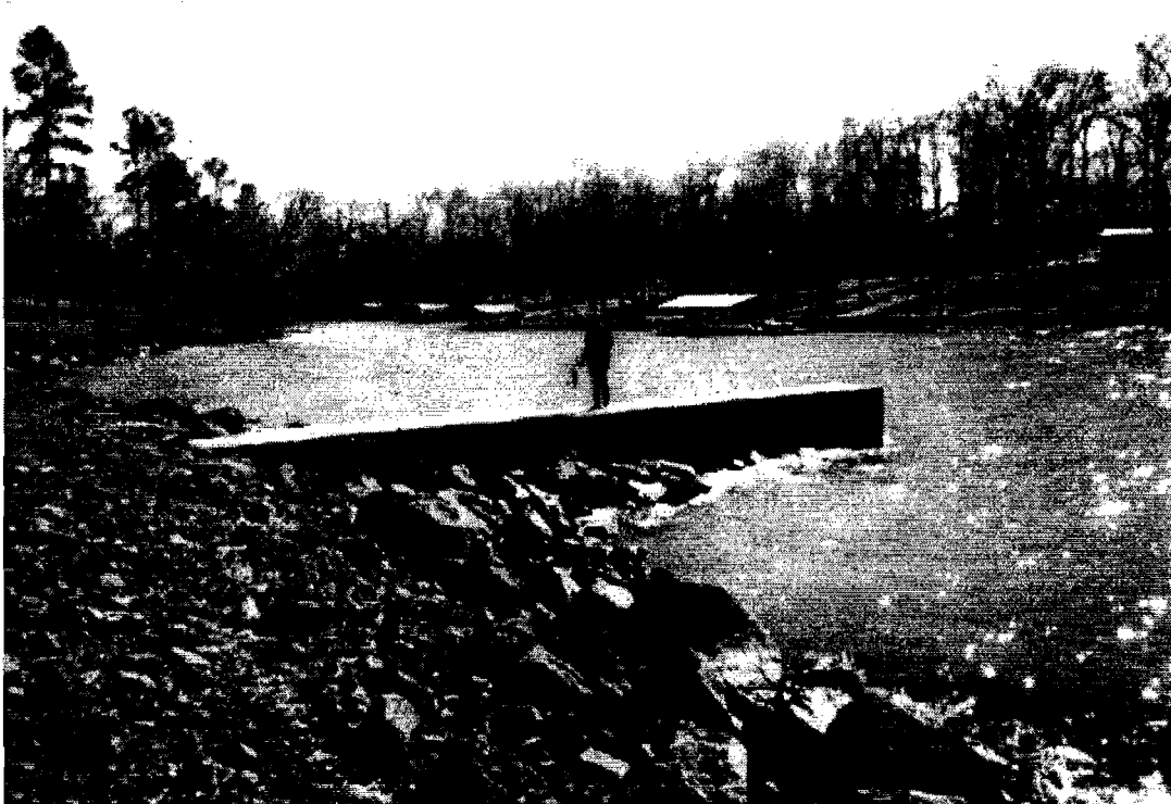
Figure 2.14: River Wing Dam Built Using Eco-Blocs (10)
