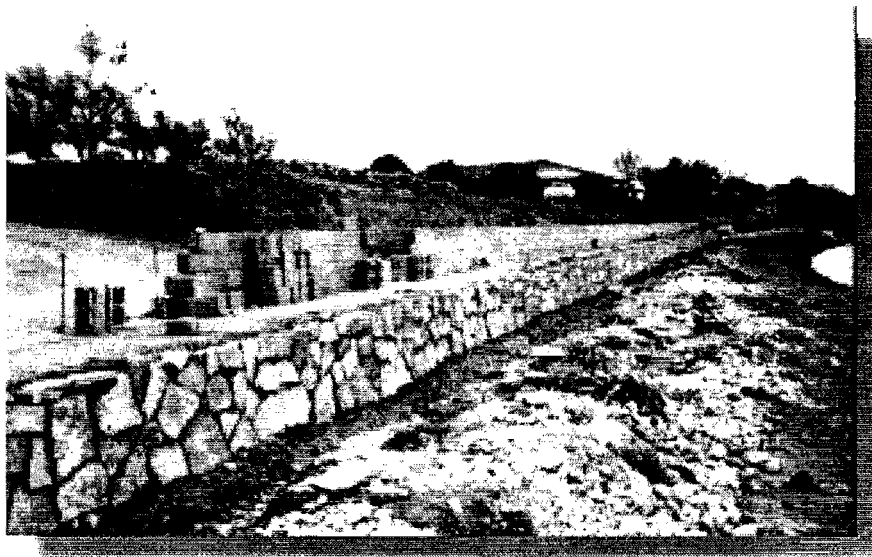
Figure 2.22: Block Retaining Wall on Top of Bales (12)
