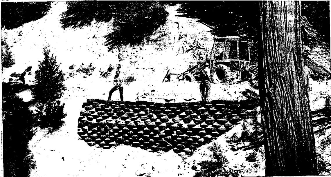
Figure 2.4. A Tire-faced Wall in California (7)
