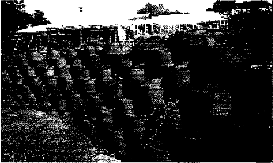
Figure 2.2. Geo-fabric used to cover the tires (8)
