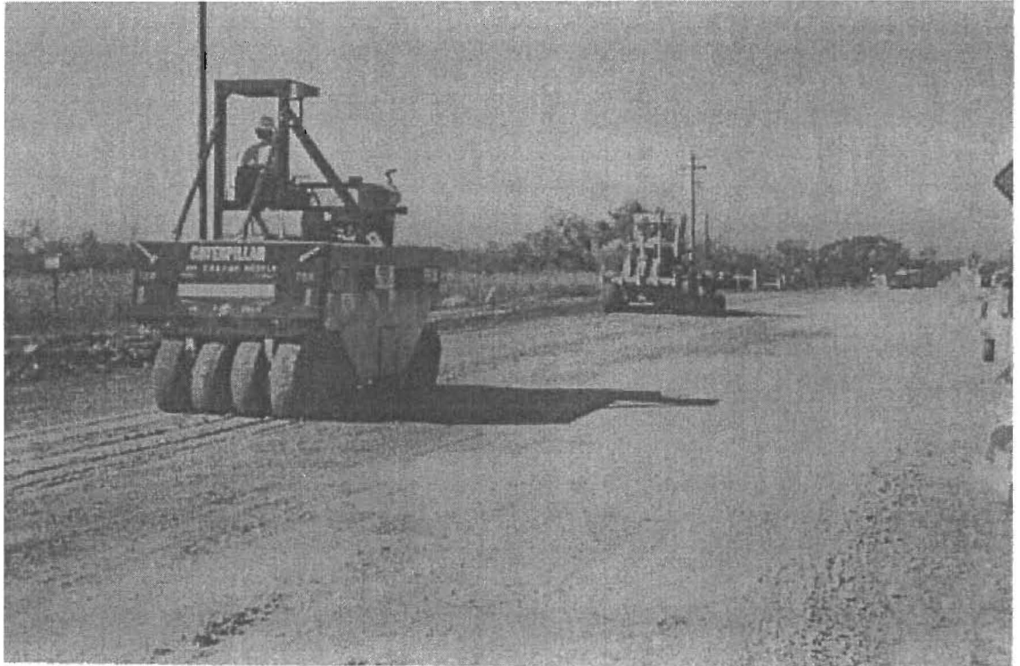
Figure 5.7: Compaction Using Pneumatic Roller.
