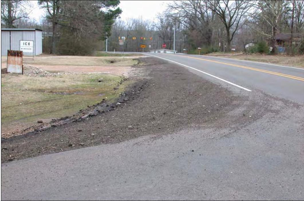
**FIG. 4.12.** Typical Edge Drop-off at Turning Radius (Maintained by placing RAP).
