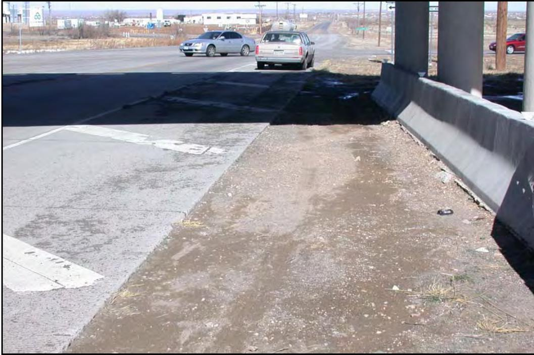
**FIG. 4.16.** Pavement Edge Damage Associated with Vehicle Pull-offs Beneath an Overpass.
