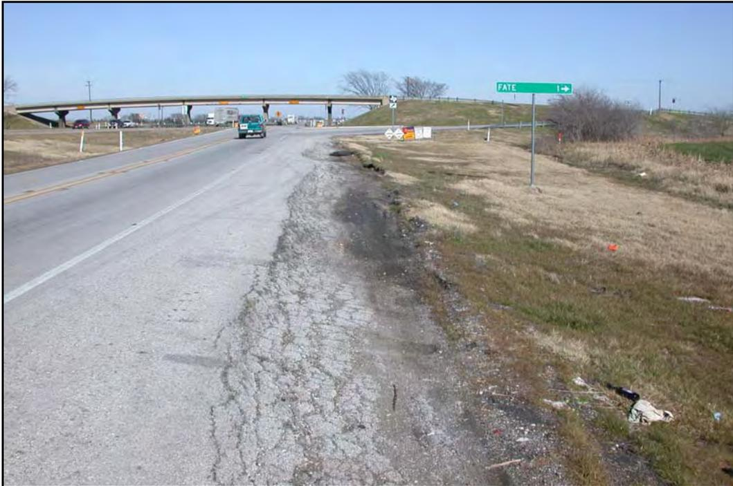
**FIG. 4.10.** Edge Damage Along Interstate Highway Access Road.
