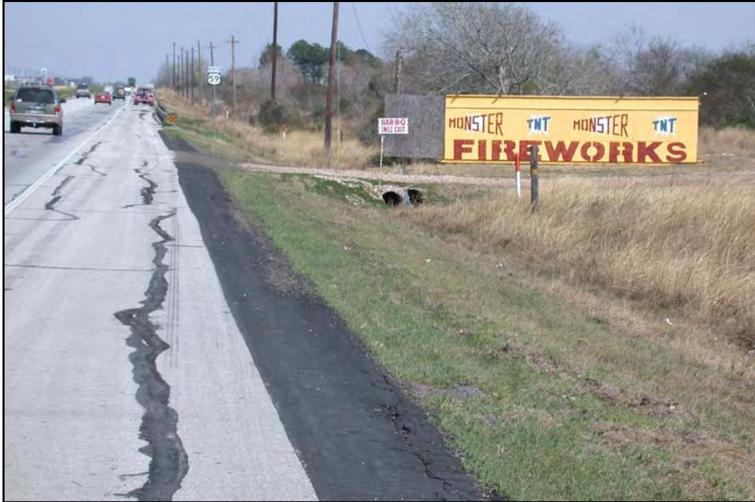
**FIG. 4.21.** Typical Edge Damage at Location of Roadside Vendor.
