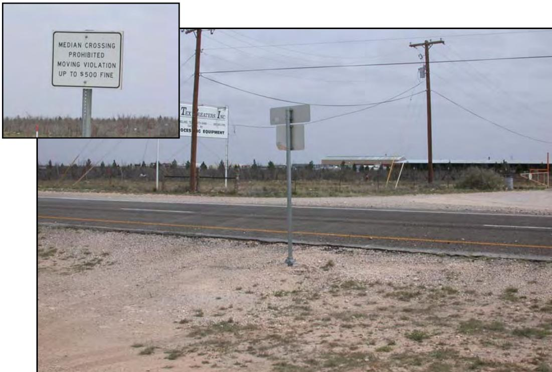
**FIG. 4.17.** Pavement Edge Damage Associated with Illegal Median Crossing. The Inset Shows the Regulation Sign Posted Where the Crossing Continues to Occur
