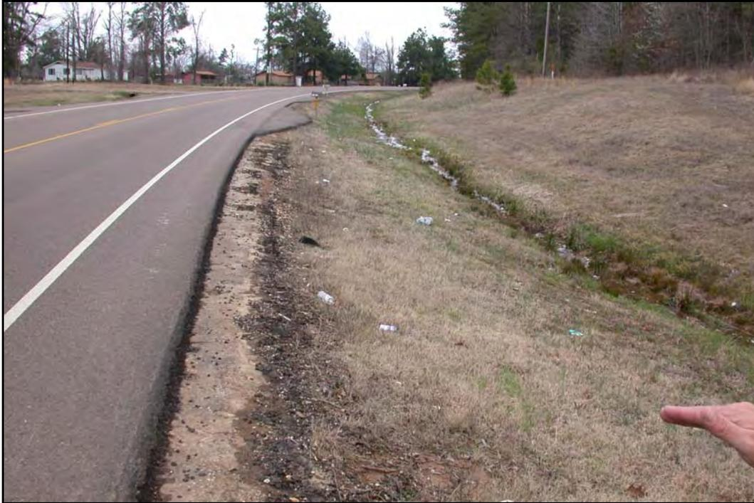
**FIG 5.13** Erosion-induced Edge Drop-off Following an Overlay, Atlanta District (see Atlanta District Profile, Photo 11)
