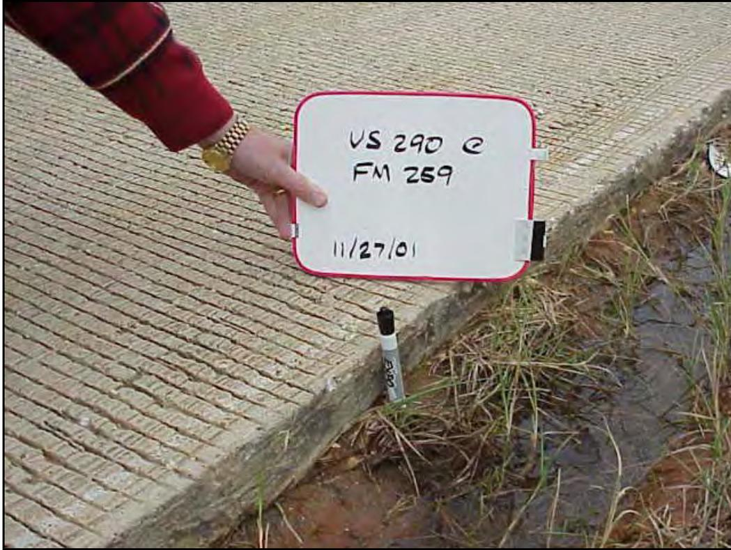
**FIG. 4.26.** Edge Drop-off Associated with Wet Subgrade Along the Edge of Pavement
