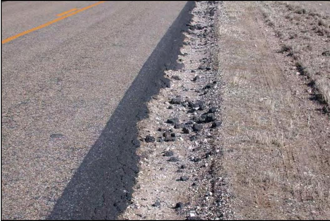
**FIG. 4.22.** Typical Edge Damage on a Low Volume Road Caused by Snow Plow Operations.
