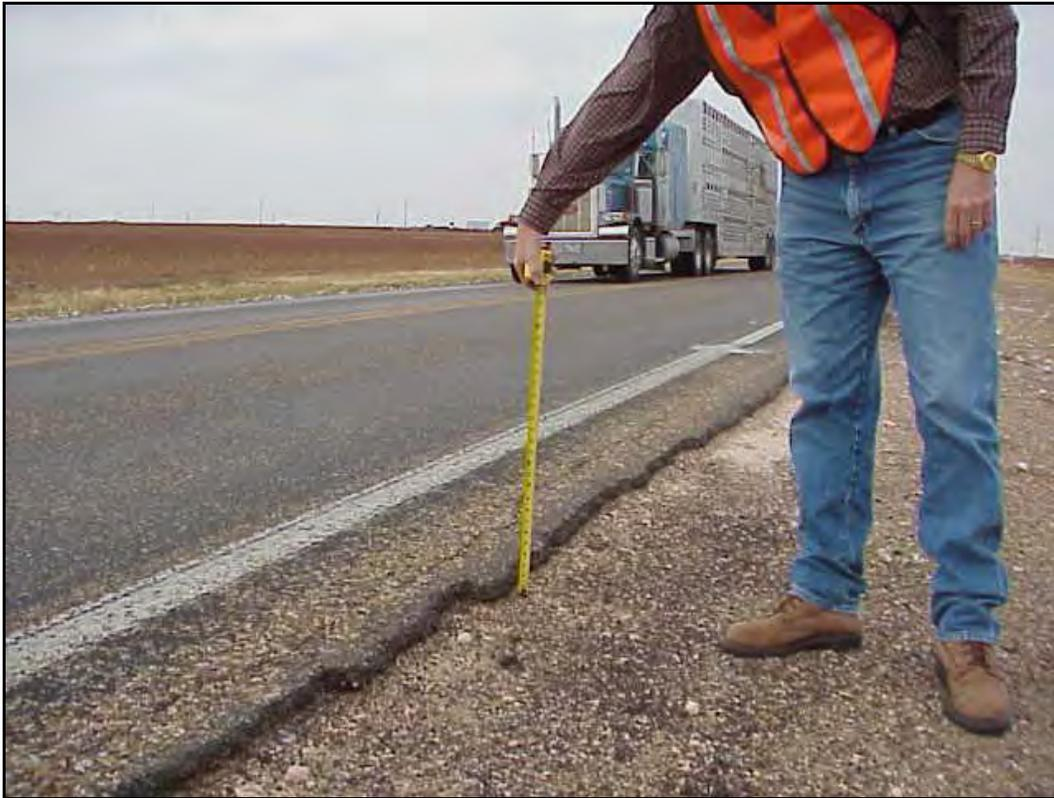
**FIG. 4.15.** Typical Pavement Edge Damage Associated with Cotton Production in West Texas.
