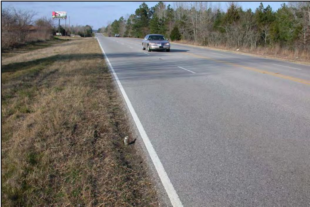
**FIG. 4.7.** Edge Drop-off Along a Narrow 4-Lane US Highway (“Poor-Boy” 4-Lane).
