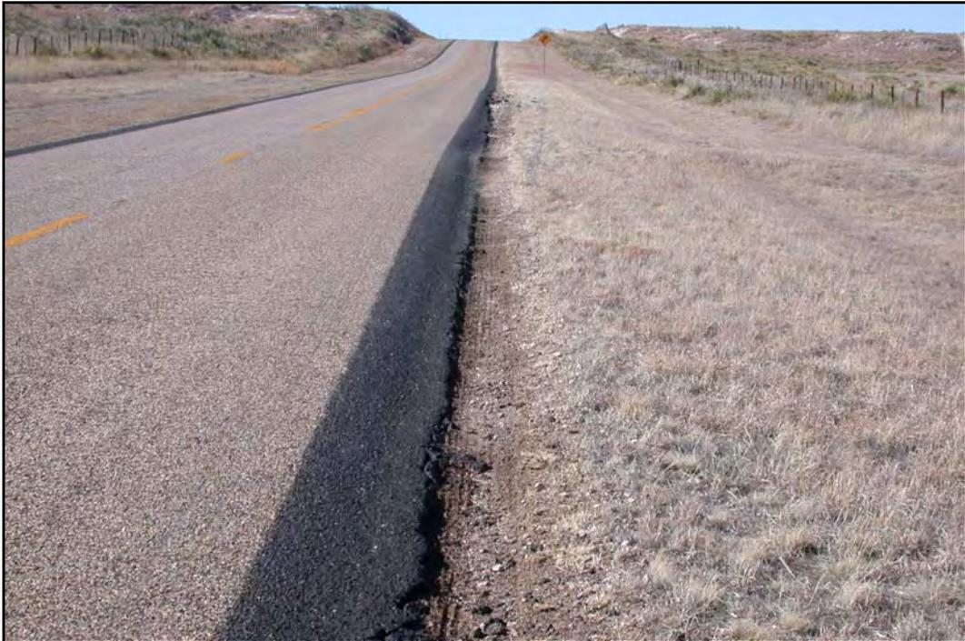
**FIG. 4.13.** Typical Edge Drop-off at Approach to Uphill Vertical Curve.
