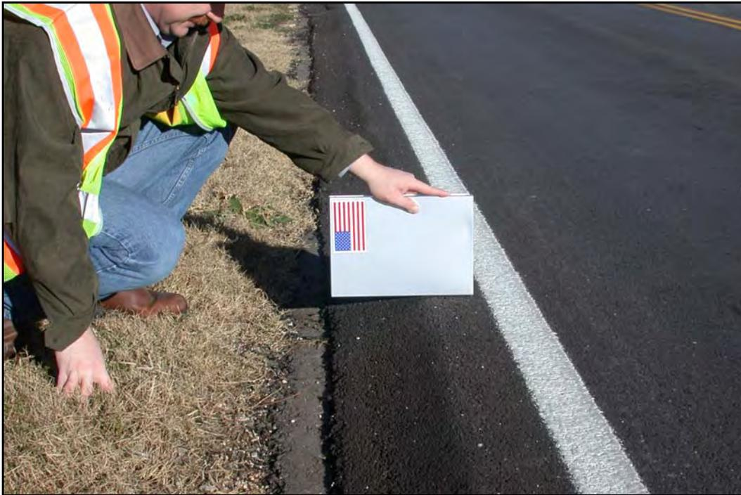
**FIG 5.5** Tapered Edge Detail to Reduce Edge Drop-offs Following a Full-Width Overlay, Fort Worth District (see Fort Worth District Profile, Photo 8)
