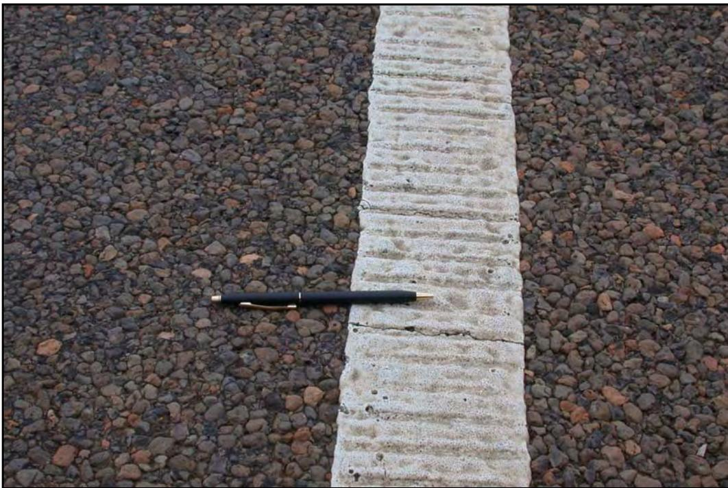
**FIG 5.21** Inverted Profile Pavement Marking, Close-up View, Atlanta District (see Atlanta District Profile, Photo 26)
