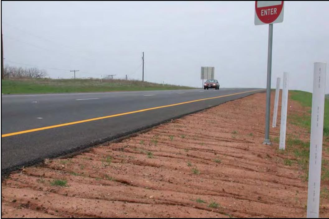
**FIG 5.6** Soil Erosion of Pavement Edge Backfill due to Improper Specification, Wichita Falls District (see Wichita Falls District Profile, Photo 7)
