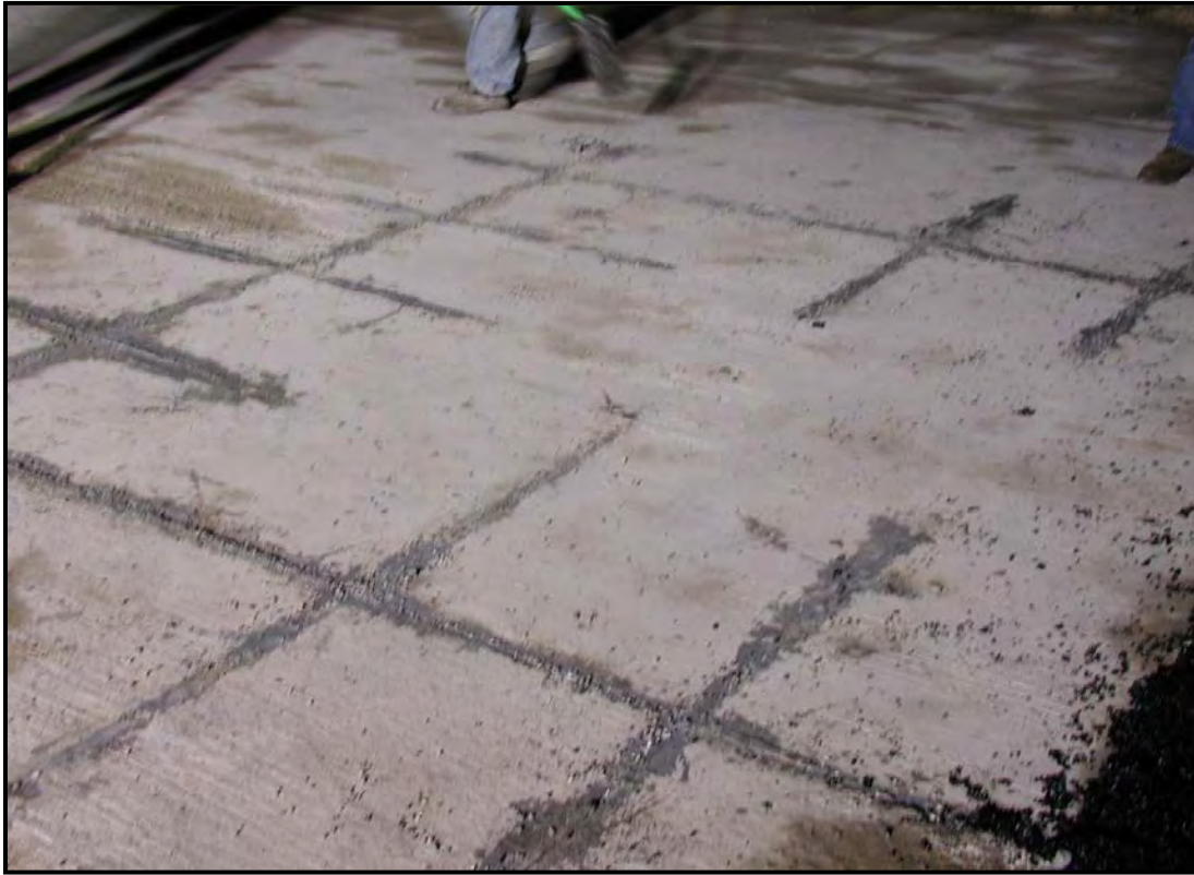
Figure 5.22 Precast Panel after the Repair has been Complete
