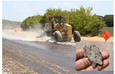
Figure 4.7 Application of Worked-In (Cut-In) Prime on Limestone Base
