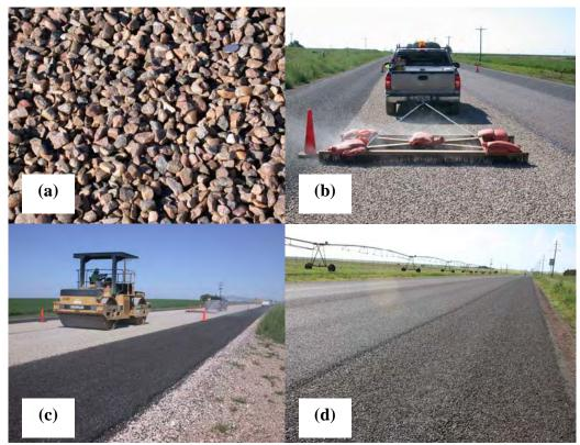
Figure 5.4 Construction of Three-Course Surface Treatment in West Texas (a) Grade 4 Rock in First Course (b) Drag Broom used for Grade 2 First Course (c) Use of Heavy Roller for Grade 2 Rock First Course (d) Edge Drop-off Between Three-Course Main Lane and Two-Course Shoulder
