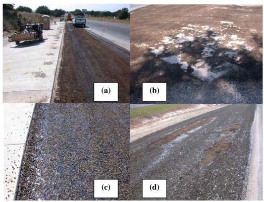
**Figure 5.9** Construction of a Surface Treatment in Texas Hill Country (a) AE-P Spray Prime Applied (b) Prime Peeled-off at Shaded Area Due to Construction Traffic (c) First Course of Surface Treatment Applied (d) Failed Surface Treatment Due to Construction Traffic
