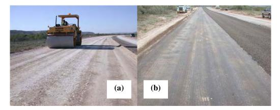
Figure 5.6 Construction of Two-Course Surface Treatment in West Texas (a) Rolling with Steel Wheel Roller (b) Second Prime Coat Applied Over First Course
