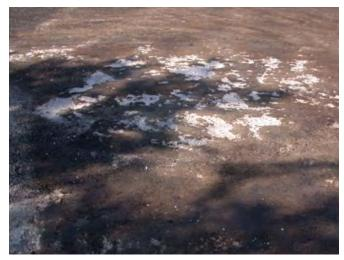
Figure 4.10 A Prime Coat That Peeled During Brooming
