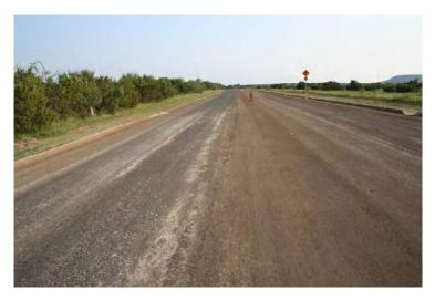
Figure 4.12 Damaged Prime Coat Due To Water-Logging
