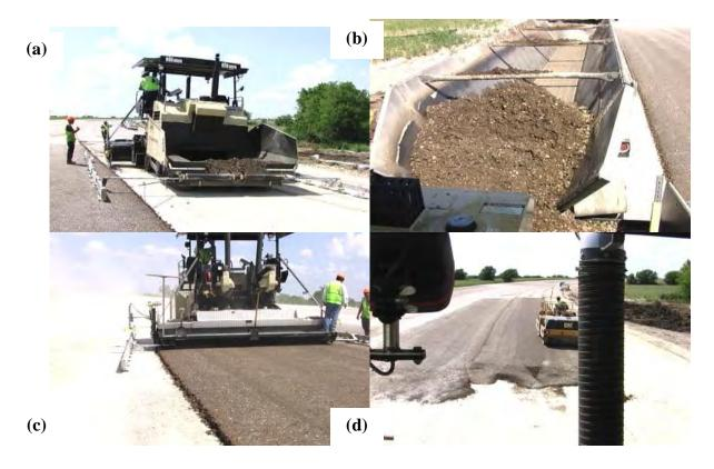
**Figure 5.10** Base Lay-Down Machine in Operation (a) Lay-down Machine and its Conveyor – Driven Hopper (b) Mixed Base Material Transported from Pugmill to Lay-Down Machine Hopper (c) Lay-Down of Emulsified Asphalt Base in Progress (d) Rolling of Laid-Down Base
