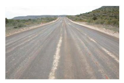
Figure 4.11 A Prime Coat Worn Out Due To Excessive Exposure To Traffic
