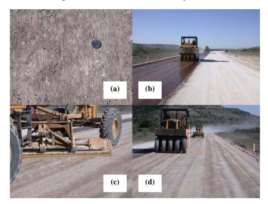
Figure 5.5 Construction of Two-Course Surface Treatment in West Texas (a) Finished Base Surface before Priming (b) MS-2 Prime Diluted 5% Emulsion/95% Water on Finished Base (c) Base Material Spread over Prime (d) Rolling with Pneumatic Roller
