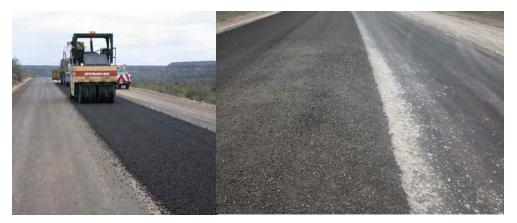
Figure 4.13 Damaged Prime Coat Due To Loose Rock
