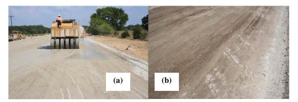
Figure 5.7 Construction of Two-Course Surface Treatment in East Texas (a) Slush Rolling (b) Bladed Surface Ready to be Primed
