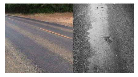
(a) (b) Figure 4.15 (a) Flushing and (b) Bleeding in Asphalt Surface Treatments
