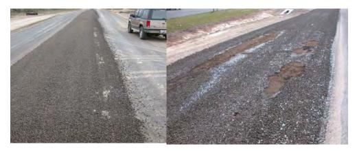
(a) (b) Figure 4.14 Peeling of Surface Treatment During Construction
