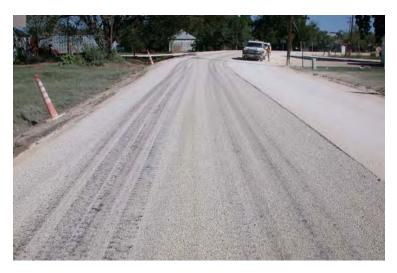
Figure 4.8 Covered (Or Inverted) Prime Using RC-250 and Grade 5 Rock
