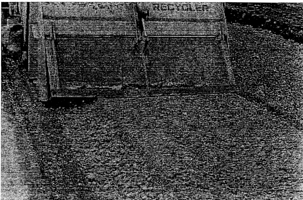
Figure 5.3. Dumping of Glass-Cullet by a Belly Dump Truck
