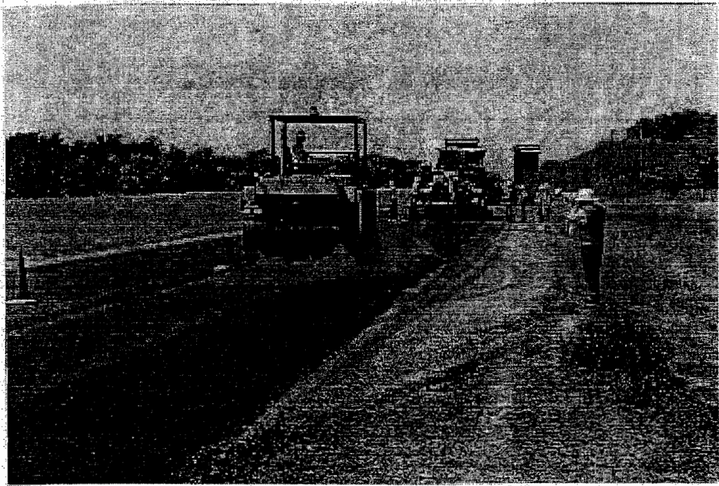
Figure 6.3. Photograph of Construction Activity on WB SH 31, Corsicana
