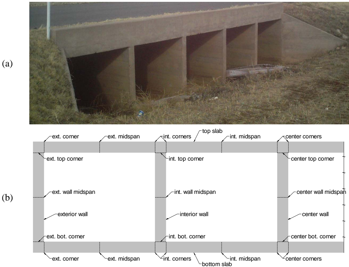
Figure 2.1. (a) A five-span reinforced concrete box culvert in Swisher Co., TX; (b) potential critical section schematic
