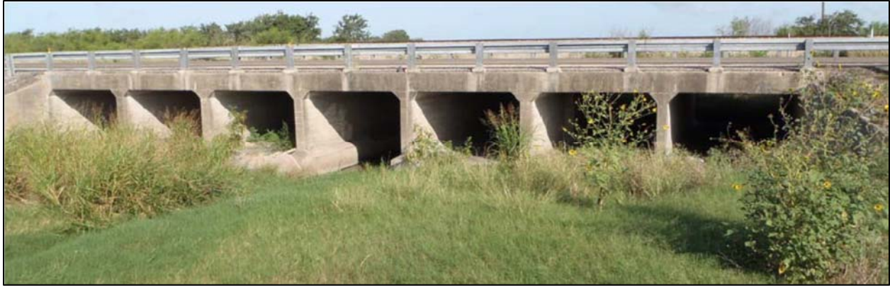
Figure 7.1 Complex 7-span reinforced concrete culvert: structure #161780010202005.
