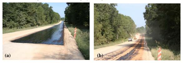
Figure 3.2 Spray Prime (a) MC-30 Cutback Prime (b) Blotting Sand Applied on Prime
