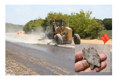
Figure 3.3 Application of worked-in (cut-in) prime on limestone base
