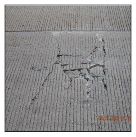
Figure 5. Partial depth distress under wheel path
