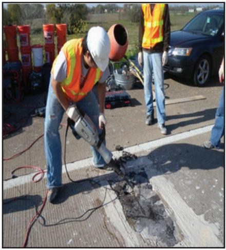
Figure 9. Removing concrete using a jackhammer
