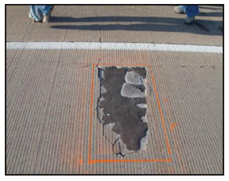
Figure 7. Boundary of PDR straight and clearly marked
