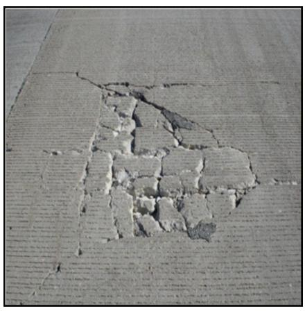
**Figure 3.** Partial depth distress under wheel path with fractured concrete
