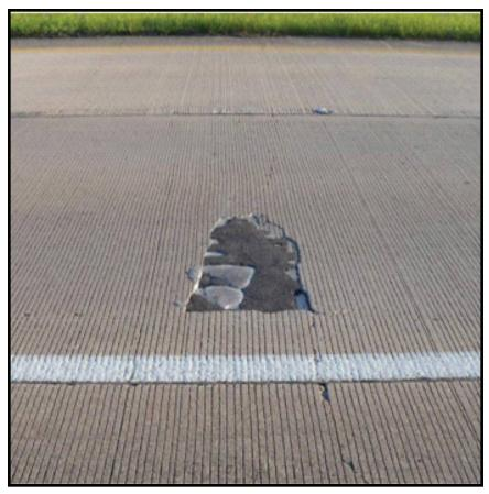
Figure 4. Partial depth distress under wheel path
