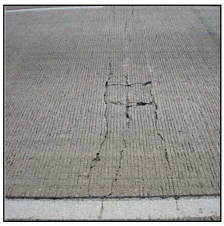
Figure 2. Partial depth distress under wheel path
