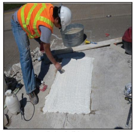
Figure 12. Application of sufficient curing compound
