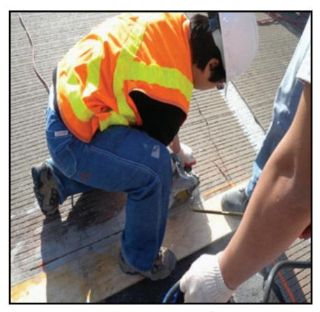
Figure 8. Saw cut operation
