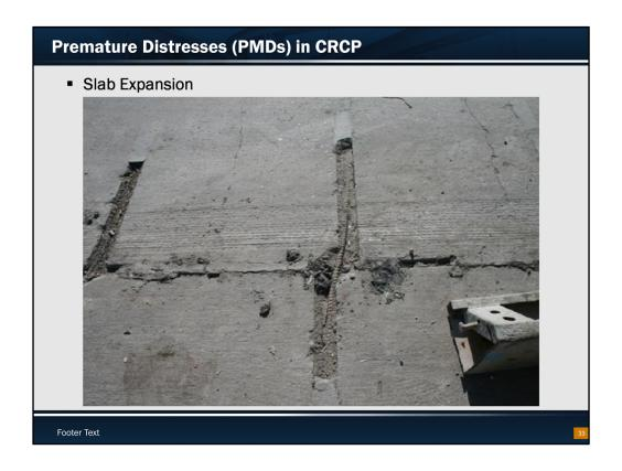
This shows slab expansion as large as 3.5 inches when the portion of the concrete in one lane was removed for pavement repair, which caused deformations in the stitching bar. The exact cause of this slab expansion is not known.
