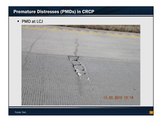
This is a distress at LCJ. It is noted that the transverse crack on the right of the distress is a normal crack in CRCP from temperature and moisture variations. On the other hand, the crack on the left has characteristics of a transverse crack due to heavy wheel loading applications. Or, it could be that there were differential displacements between the two lanes, which could have caused minor damage to the concrete in the outside lane.
