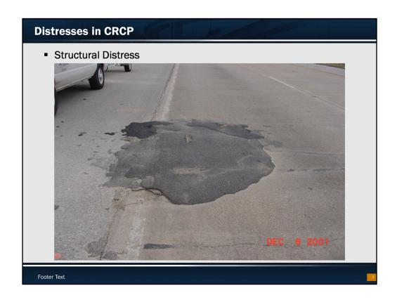
The distress shown in this slide is covered with asphalt and the mechanism of this distress is not easy to identify. However, based on the area and location of the distress, it is considered as a structural distress.
