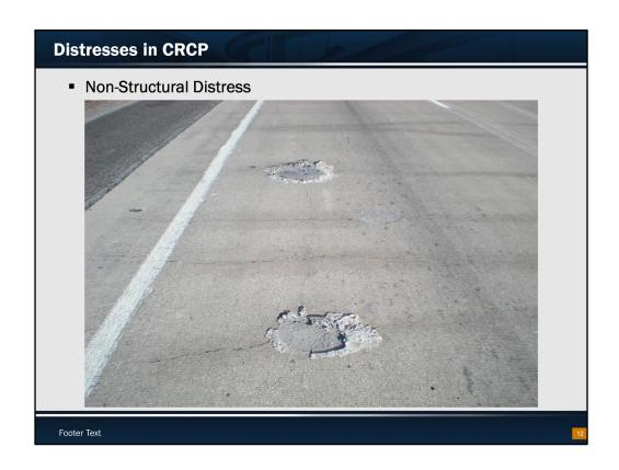
Spalling with longitudinal cracking. It appears that wheel loading applications at locations with transverse and longitudinal cracks resulted in spalling. Spalling in this project was quite rare, and it is considered that the quality of construction was a cause for this distress.
