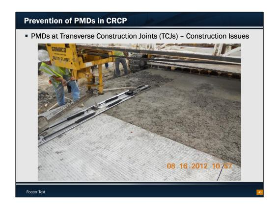
This shows the auto-float operation at a TCJ. Note the surface condition of the concrete. The rough surface condition is due to the hand operations of concrete placement near a TCJ. This rough surface will be smoothed by excessive floating, which may not be able to remove all the voids in concrete.
