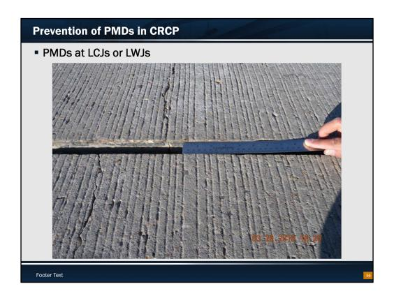
This slide shows a differential slab movement in the longitudinal direction as large as 1 in at LWJ between two lanes. Since the same concrete materials were used in this project, the large differential slab movements appear to be due to the instability in the base/subgrade layers. In this slide, lane separation is also noted, which further indicates volume changes in the layers below the concrete slab.
