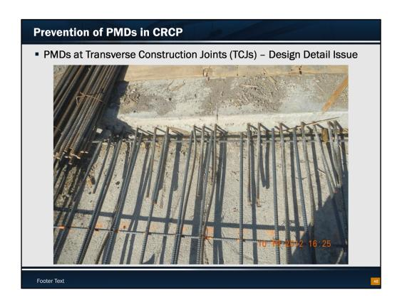
This shows the steel placed at a TCJ. It is observed that steel is somewhat crowded and extra effort should be made to ensure good concrete consolidation.
