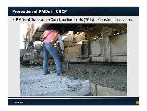
This illustrates consolidation of concrete at a TCJ by a hand vibrator, which is again different from consolidation operations in the other areas where a paver with mechanical vibrators consolidates the concrete.
