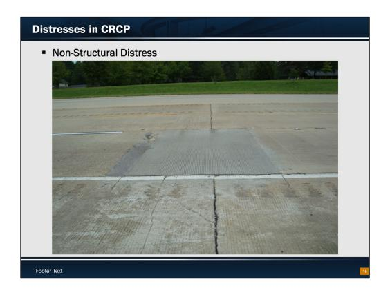
This shows a repair of distress at a TCJ. It is reported that additional longitudinal tie bars at TCJs in southbound lanes were placed at every spacing between longitudinal bars, i.e., double the required amount. Additional tie bars for the construction of northbound lanes were in accordance with the requirements in the design standards, and no distresses were observed. This case illustrates that doubling additional tie bars at TCJs is not a good practice.
