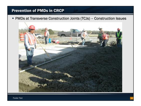
This shows finishing operations at a TCJ. Note that a slip form paver placed the concrete, but with no surface finishing operation, which is done by hand operations. Hand operations are not effective in removing all the voids from concrete. Field evaluations of concrete near TCJs indicate voids in concrete near the surface, degrading the durability of the concrete.
