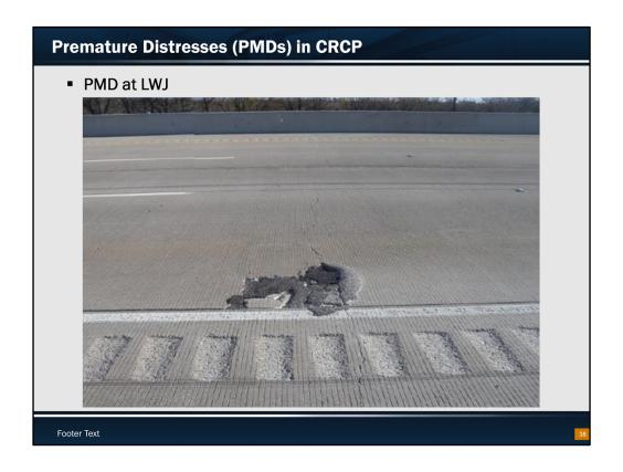
This shows a distress at LWJ. It is noted that the distress is not only near the LWJ, but under the wheel path as well. In other words, it could be that slight damage to concrete from differential movements transmitted by transverse steel and tie bars at LWJ occurred first, and subsequent wheel loading applications could have caused the distress.
