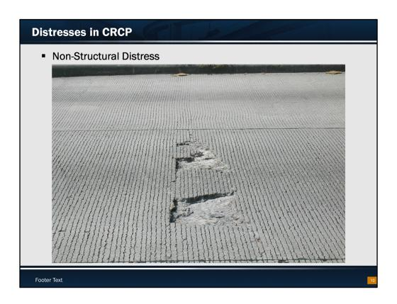
This distress shows a typical spalling due to the use of a specific coarse aggregate type, whose coefficient of thermal expansion is larger than other aggregate types.
