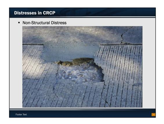
Another spalling distress in severe condition. Shallow delamination is observed. This section was placed in the winter in Houston when the concrete placement temperature was ideal. This distress indicates "temperature control" during concrete placement is not effective in reducing the spalling potential of concrete containing coarse aggregates prone to spalling.
