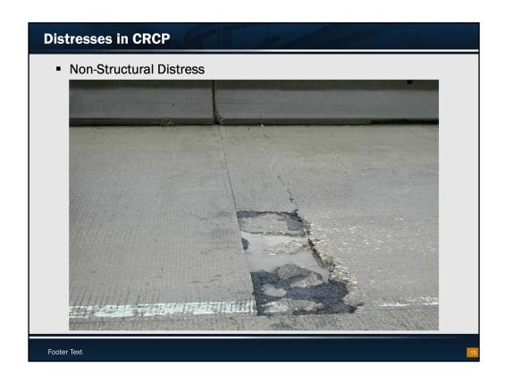
Typical shape of a distress at a transverse construction joint (TCJ). A transverse crack next to the TCJ coincides with the end of additional longitudinal tie bars. This distress is not structural capacity related; rather, it appears to have to do with TCJ.
