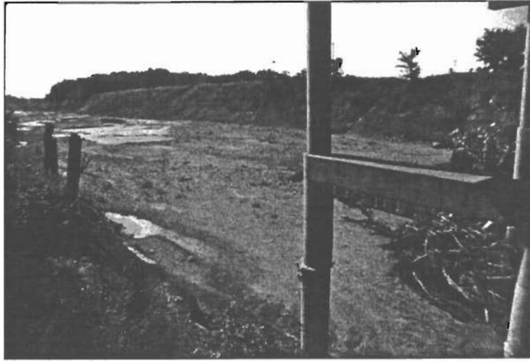
Figure 19. This is a view looking upstream from the FM 2990 bridge crossing the North Sulfur River in Fannin County. In response to the straightening of the Sulfur River Channel, dramatic lowering of the channel bed by regional down cutting has occurred. The drop in channel bed elevation was caused by the artificial straightening of this reach of channel that resulted in the steepening of gradient. The ring shown on the concrete pier shows the level of the channel when the pier was poured.
