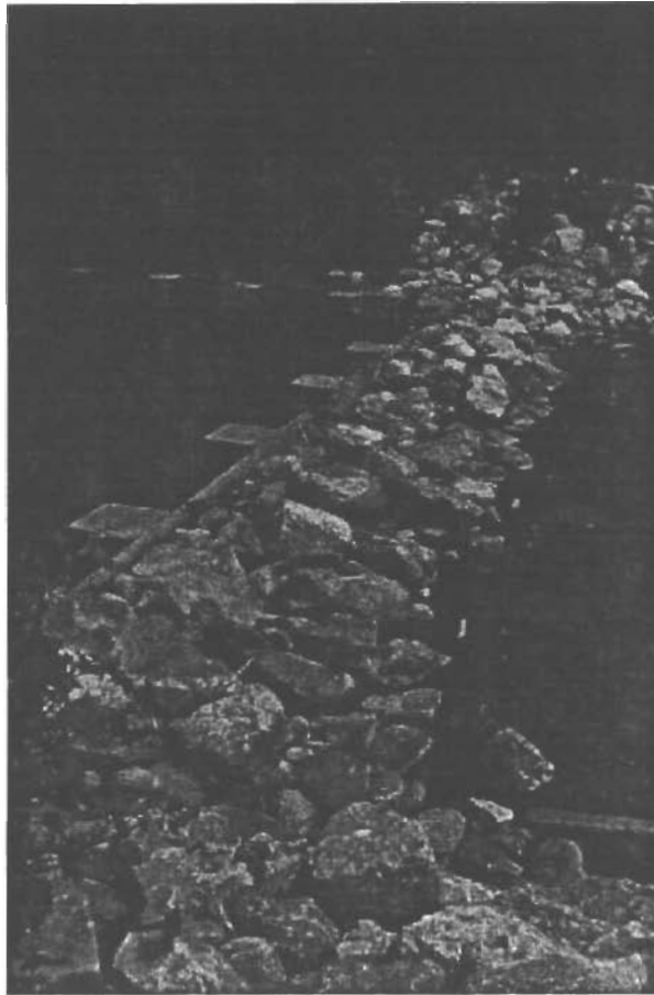
Figure 16. Downstream side of the grade control structure.
