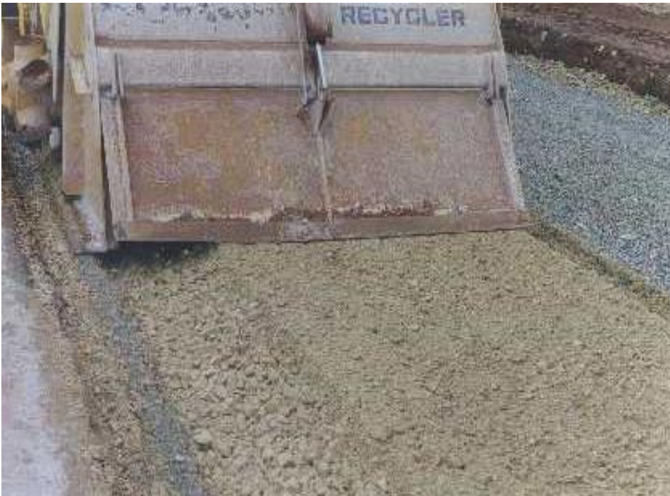
Figure 2. Mixing of glass cullet with limestone in Abilene District
