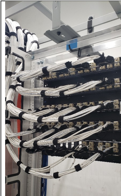
Back of patch-panel showing cables routed to vertical management.
